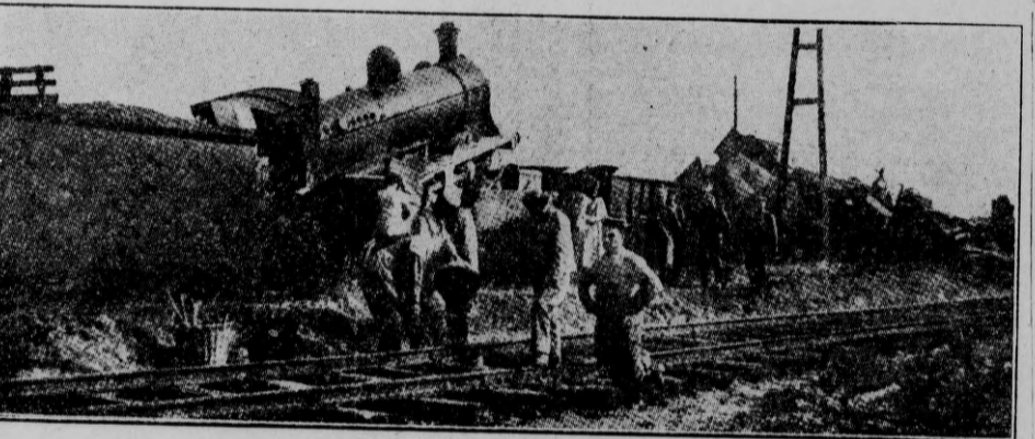
The havoc made by the locomotive charge mentioned above was so great that the Germans found it more expeditious to build a new track parallel with the old one instead of attempting to remove the wrecks and repair the old line.
